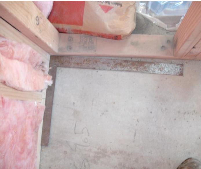
Walls built out of square
