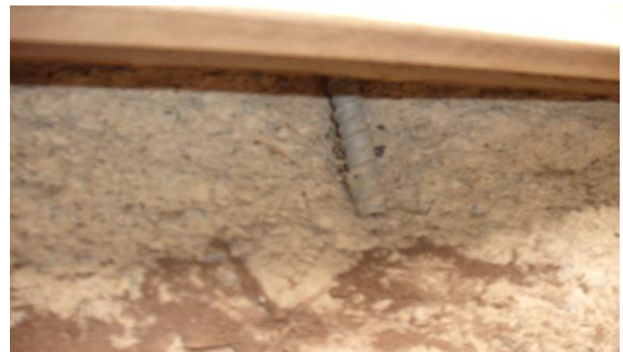
Multiple hold downs through slab edge across tow building elevations
