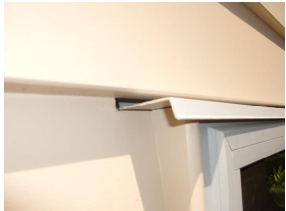
Head flashing with slope toward building
