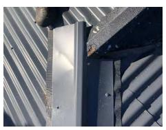
A raised valley placed over the top of the existing valley. No valley purlins were installed with the roof over existing tile battens.
