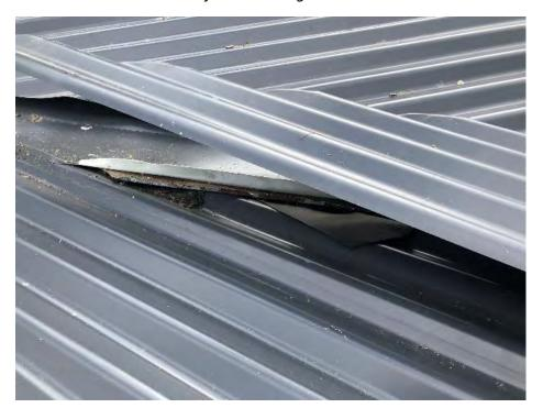
New roofing layed over existing tile battens. Purlins have been installed on the bottom row & ridge/hip rows. The purlins are thicker than the battens & damage can be seen on a lot of the sheets from this.
