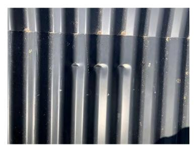
The sheeting behind the chimneys is appalling. As corrugate has an overlap & an underlap to sheet behind a chimney this way involves creating an overlap out of an underlap. This needs to be marked & cut carefully but will never be as good as a factory edge. There has been one attempted to achieve this & the cut is poor. Other sheeting behind the chimneys has the overlap left uncut. Silicon has been applied to one to prevent water entering inside.
