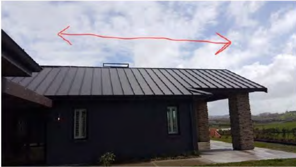
Area where the ridging blew off the roof on 22 August 2019
