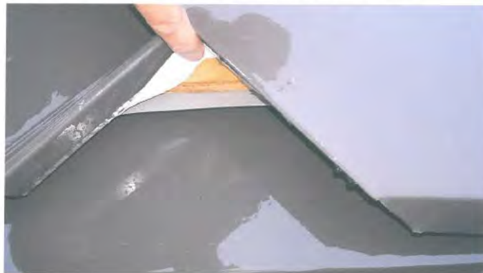
Hole in roof as installed by Tactical Roofing – photos supplied by builder Nick Paterson
