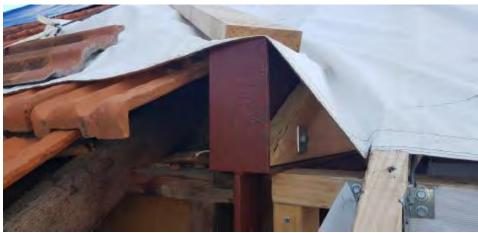
[34] With regards to the minor dwelling trusses have been made to the incorrect roof pitch and height setting. Truss members have been cut and altered on site to try and align with the existing roof. This has caused additional issues with the eave overhang then not lining up. The Respondent stated that he was not on site when the trusses were measured. The Complainant stated that the minor dwelling has had the
