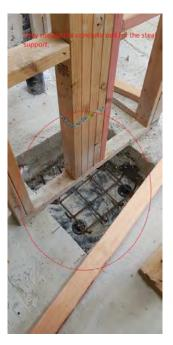
[25] A structural column to the blockwork wall was missed, requiring the blockwork to be cut to allow the reinforcing to be placed so that the column could be formed. The engineer's pre-pour site inspection required reinforcing to be placed as per design. As this had not been done he required vertical bars to be epoxied into the concrete slab as shown in photograph below:
