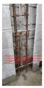
[26] The concrete did not go all the way down nor was every cavity filled. The Engineer was required to re-inspect the blockwork. The blockwork wall was scanned, and the unfilled cores were re-filled under instruction. The photograph below depicts the work.
