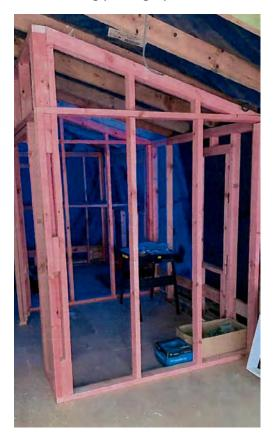
(e) Master bedroom dormer roof was not constructed in accordance with the Building Consent and NZS3604:2011. Continuous rafters have been cut at the top plate line, as shown in the following photograph:
